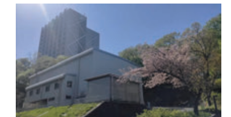
The new TSUBAME 4.0 data center on the Institute of Science Tokyo's Suzukakedai Campus
