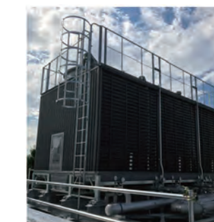
Free cooling tower producing cooling water at near outdoor temperatures
